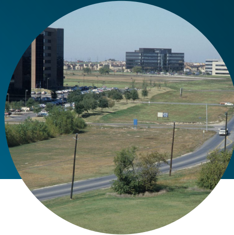
Dallas North Tollway
