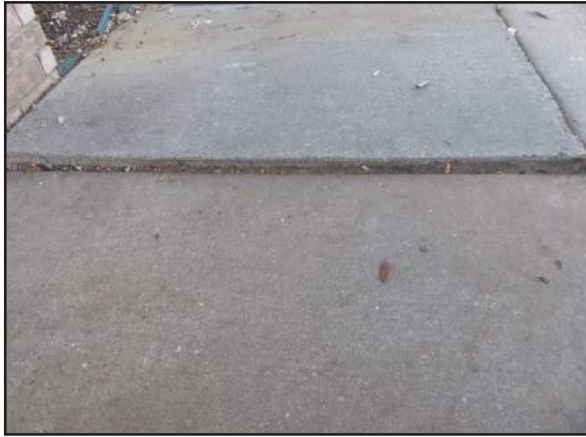
Figure 9-6 Offset – 1 Inch or Greater Example
