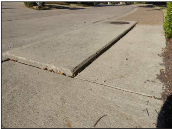
Figure 9-8 Offset – Storm Drain Inlet Example
