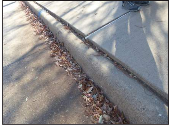
Figure 9-7 Uplift Example
