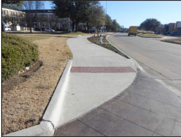
Figure 8-2 Curb Ramp Example #1
