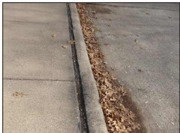
Figure 9-11 Separation Example
