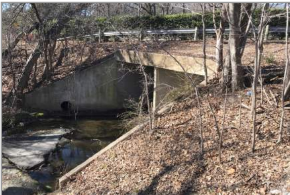
Figure 7-7 Substructure – Double End Wall
