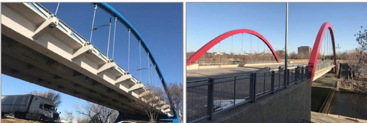
Figure 7-3 Superstructure – Arch, Support Cable
