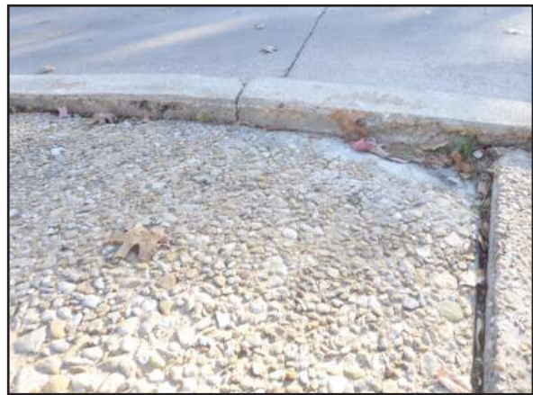
Figure 9-9 Depression Example
