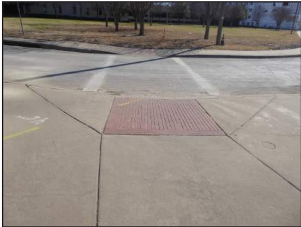
Figure 8-5 Curb Ramp Example #4
