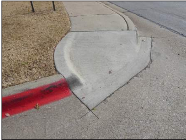
Figure 8-3 Curb Ramp Example #2
