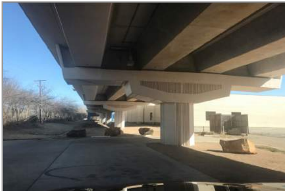
Figure 7-8 Substructure – Box Girder
