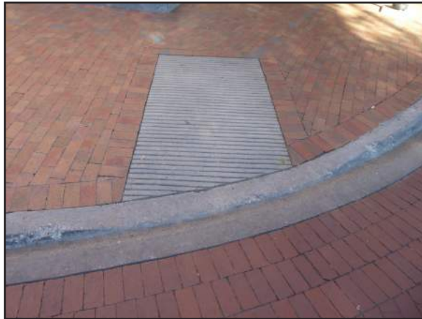
Figure 8-4 Curb Ramp Example #3
