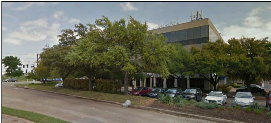
Bank and office building on Beltway at Belt Line
