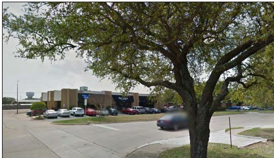
Office building on Beltway
