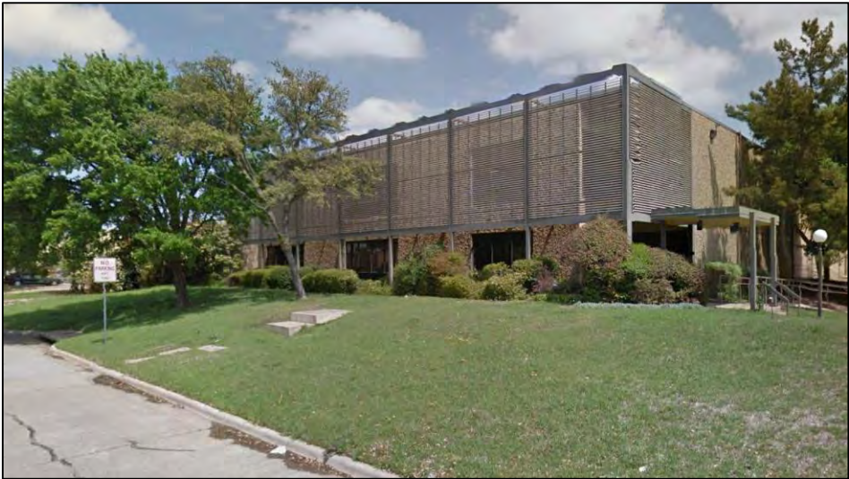
Office/light industrial building on Beltwood
