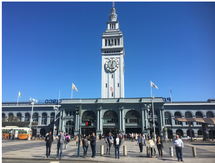
San Francisco Ferry Building Marketplace: Historic ferry port and transit hub restored with shops oriented toward local farmers and artisan food producers
