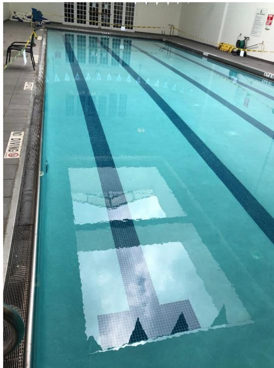
Less than a month ago, the Town started the indoor pool resurfacing project at the Athletic Club. Over the past three weeks, contractors have removed the old pool plaster and replastered the pool with Diamond Bright plaster, re-grouted the tile lane lines and targets, cleaned and polished the stainless steel gutter, and installed both new LED underwater lights and new depth markers and no diving decals.
