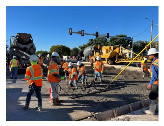
On Saturday, November 13, **Belt Line Road will be reduced to one lane in each direction** at Midway Road from 7am until about 5pm to allow concrete trucks to deliver concrete for this phase of the intersection reconstruction.
