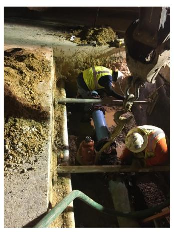
Utility work continues on the Midway Road Revitalization Project at the Belt Line/Midway intersection and from Hornet Drive to Proton Road. Over the next few weeks, crews will be replacing the large waterline valves in the intersection and installing new waterlines across Belt Line Road. This work is being completed in phases to minimize the impact on area businesses as much as possible.
