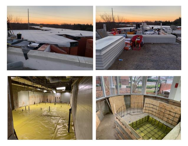
Phase One demolition at the Athletic Club is largely complete and the new plumbing, electrical, and structural work is underway for the locker rooms, pools, and hot tub. As is anticipated with any renovation project on a building of this size and age, demolition revealed existing conditions in hidden spaces (inside walls and under the foundation) that have to be addressed. These include the need to replace wood and other structural
