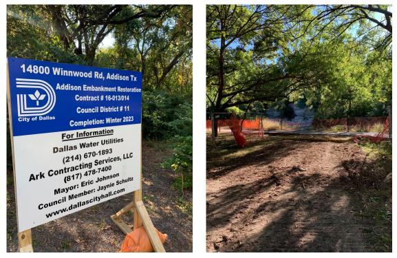
Dallas Water Utilities (DWU) began work earlier this month installing of 150 linear feet of gabion baskets along the White Rock Creek embankment and restoring the turf and trail damaged during its water line leak repair in February. The work is scheduled to be completed in February 2023.
