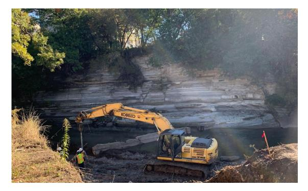
Dallas Water Utilities (DWU) is in the process of drilling the anchors for the gabion baskets that they will install along the White Rock Creek embankment. They are on schedule to complete repairs and restore the turf and trail damaged during its water line leak repair by the end of February 2023.
