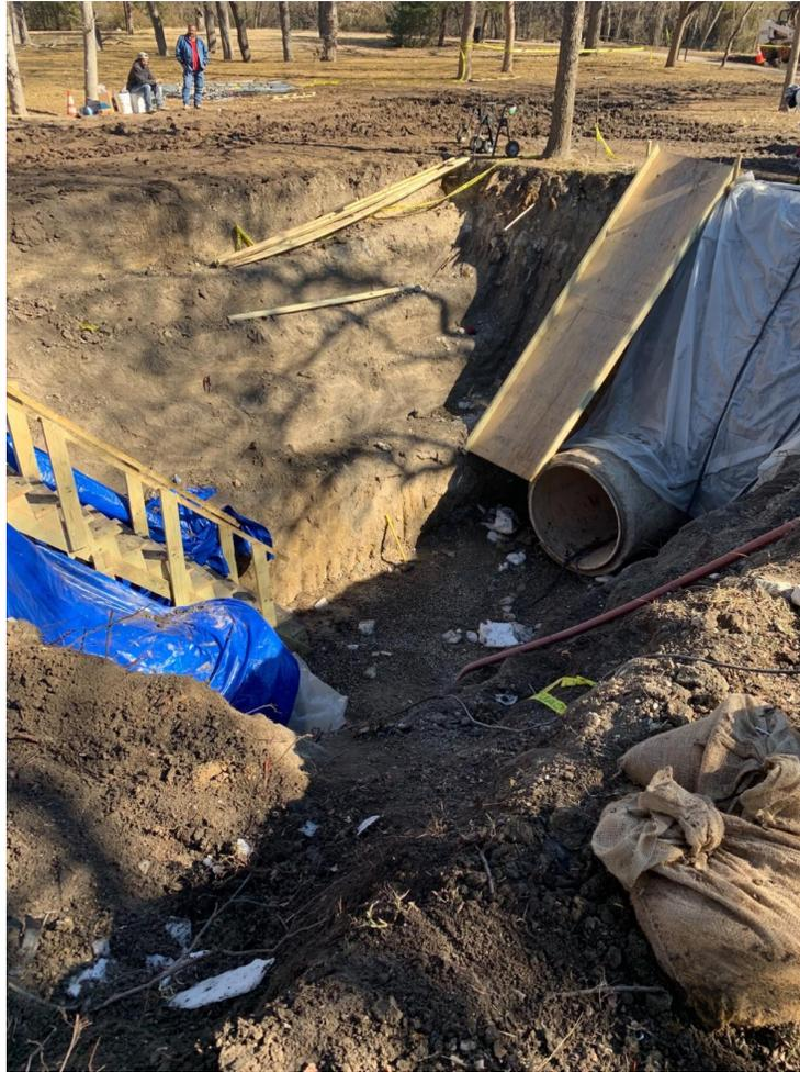
The team at Dallas Water Utilities (DWU) has been working around the clock to repair the broken water line that runs along White Rock Creek. They have completed the repair, were inspecting the line this week, and then will install the section of pipe that they had to remove to reach the break. Once that installation is finished, they can finally backfill the hole.
