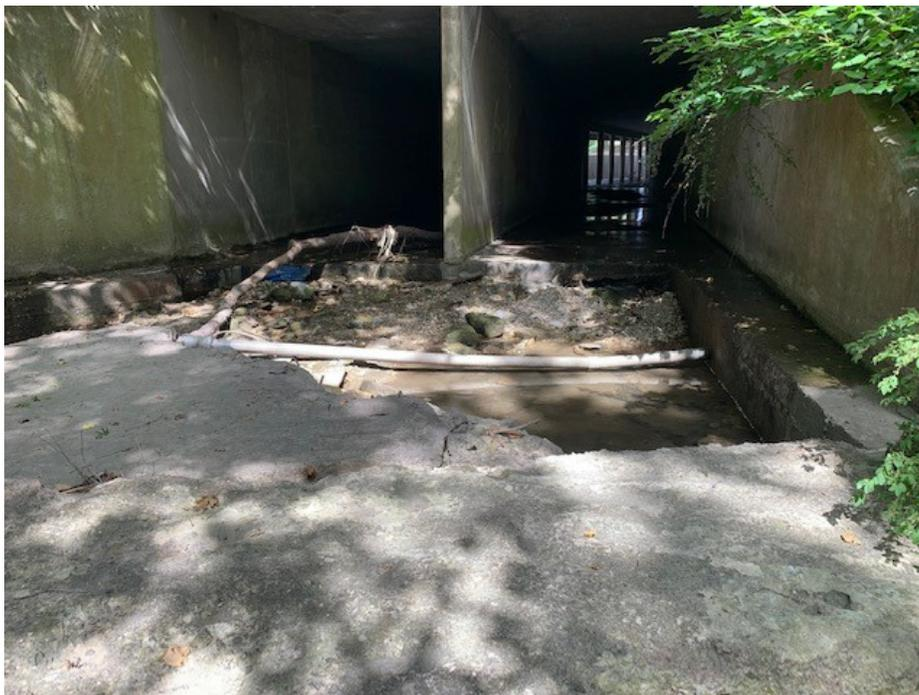
Later this month, Addison Public Works will begin construction to repair/rehabilitate the existing Winnwood Road Bridge drainage outfall to prevent future damage to the bridge due to potential erosion issues.
