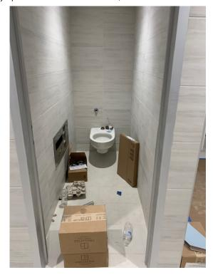
There is light at the end of the tunnel for the Athletic Club Renovation Project! Over the last two weeks, there has been a lot of tile being installed in both the lobby and locker rooms. The locker room toilets are also being installed.
