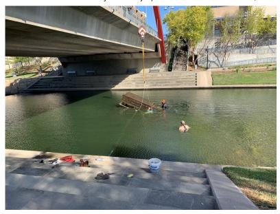
Crews were out on Wednesday, July 6 to remove the water recirculation and fountain pumps at Vitruvian Pond for repairs. All underwater repairs have been completed, and above-water electrical repair work is underway.
