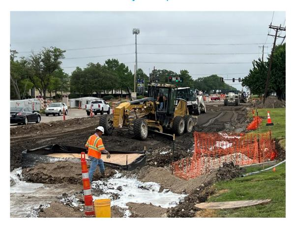
Now that the rain is over, the grading crews have moved back in to complete the grading on the west (southbound) side of Midway Road from Spring Valley Road to Proton Drive. Next week the subgrade stabilization crew will start the Lime Stabilization process and placement of Main Lane Paving is scheduled to start in two to three weeks.
