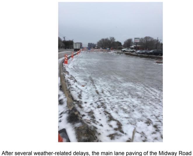
Revitalization Project from Belt Line Road to Proton Drive is scheduled to begin the week of February 13. Activities will include the fine grading and lime stabilization of the subgrade, installation of the reinforcing steel and joints, and finally the placement of the street pavement. Franchise and private utility adjustments and sidewalk, trail, and accessible ramp
