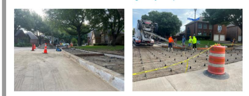
The contractor on the Rawhide Creek Basin Drainage and ADA Improvements is making remarkable progress on the project. All storm sewer pipes have been successfully installed, and the restoration of the street pavement is swiftly underway. We anticipate finishing the entire street pavement within the next two weeks. Once this milestone is achieved, the contractor will install the storm trap system adjacent to Marsh Lane and commence landscaping and restoration efforts.
