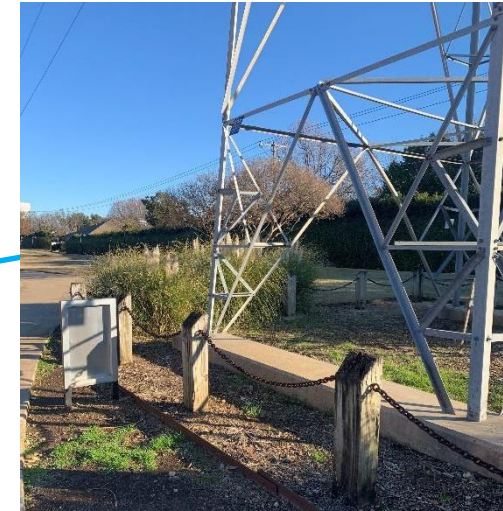
Structure Zone - Requires a 25 Foot perimeter from tower base. Turf Planting Only.
