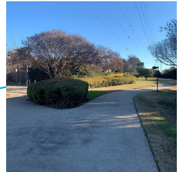
Vegetation in path of construction.
