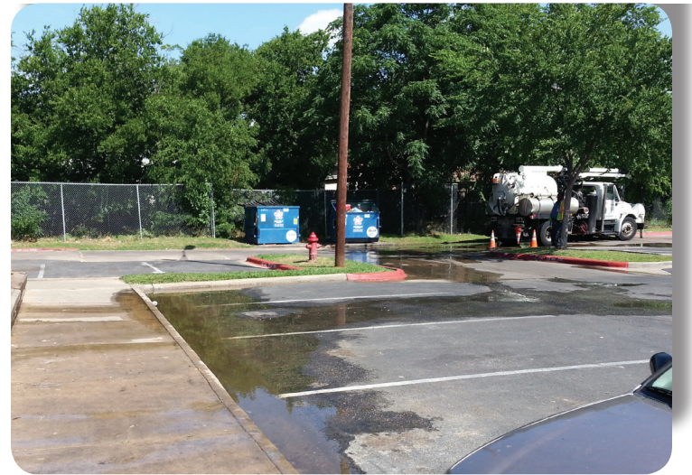
Sewage overflows are a threat to human health and can negatively impact to the value of your property.
