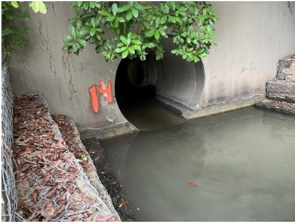
Outfall #15: 72" RCP that discharges to White Rock Creek Tributary 1.
