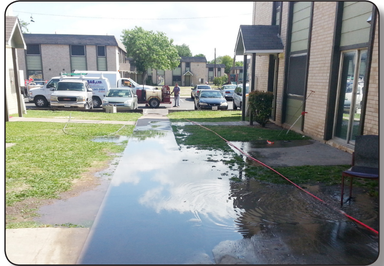
Sewage overflow at an apartment complex.
