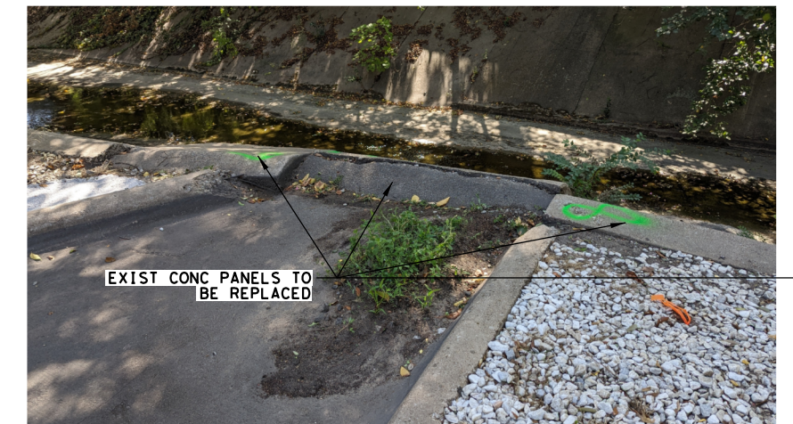
EXHIBIT 3: LOOKING SOUTH FROM OUTSIDE THE CHANNEL
